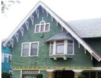
The large gable roof with rafters and fascia detail distinguishes this home as a Craftsman.
