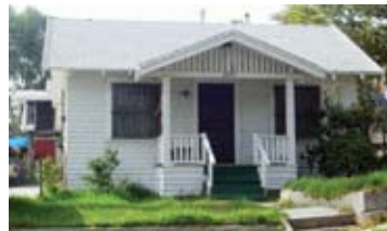
The decorative details in this all-white house are not visible. Painting it in two or more colors will make the features stand out.
