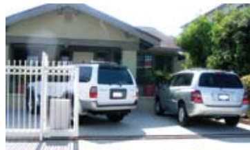
The concrete front yard with a tall fence gives this historic property a hard, unwelcoming look.
