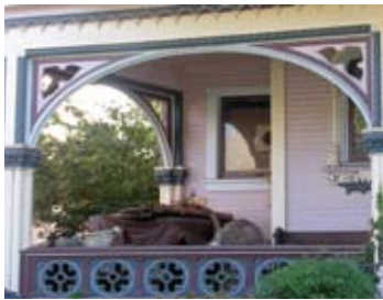
This late Victorian/Queen Anne porch has interesting and intricate detail.
