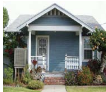
The central door opening has been filled-in & a new door has been placed off-center.
