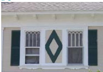
The trim and true-divided light double-hung windows are functional and decorative.
