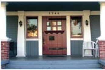
This wide door with square panes of glass & sidelights is typical of Craftsman architecture.
