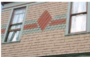
The decorative detail of the wood shingles has been preserved, and highlighted by change in color.
